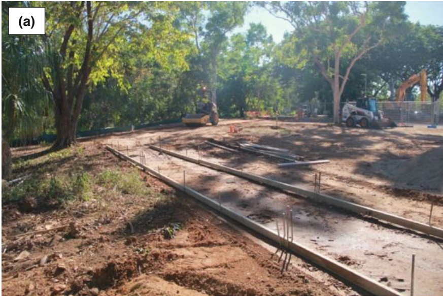
Footpath form work and a road roller compacting the soil base
