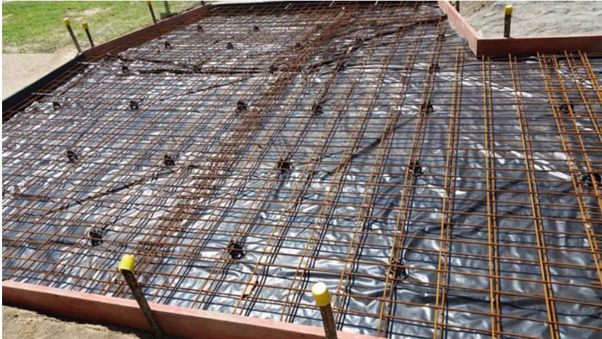
Fig. 7.1 Steel reinforcing mesh for concrete footpath
