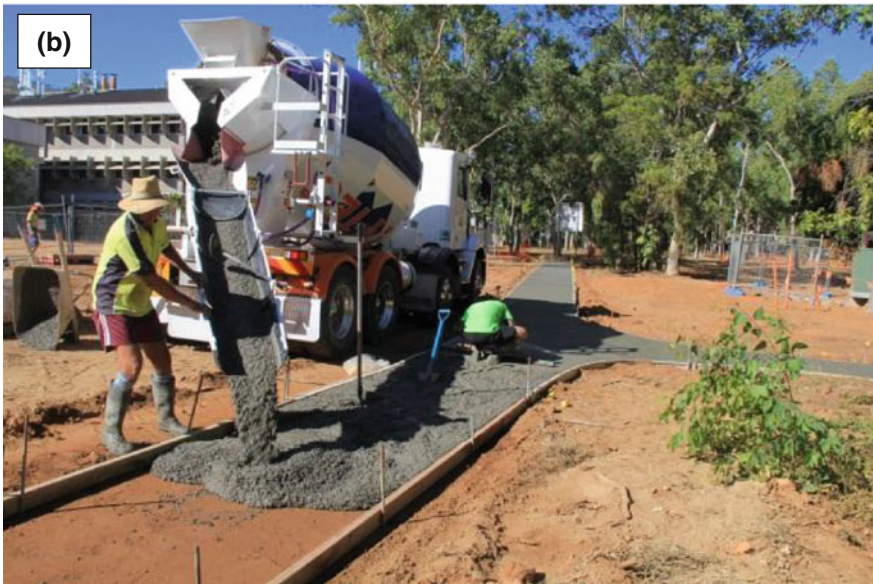
Ready-mixed concrete pouring into the form work
