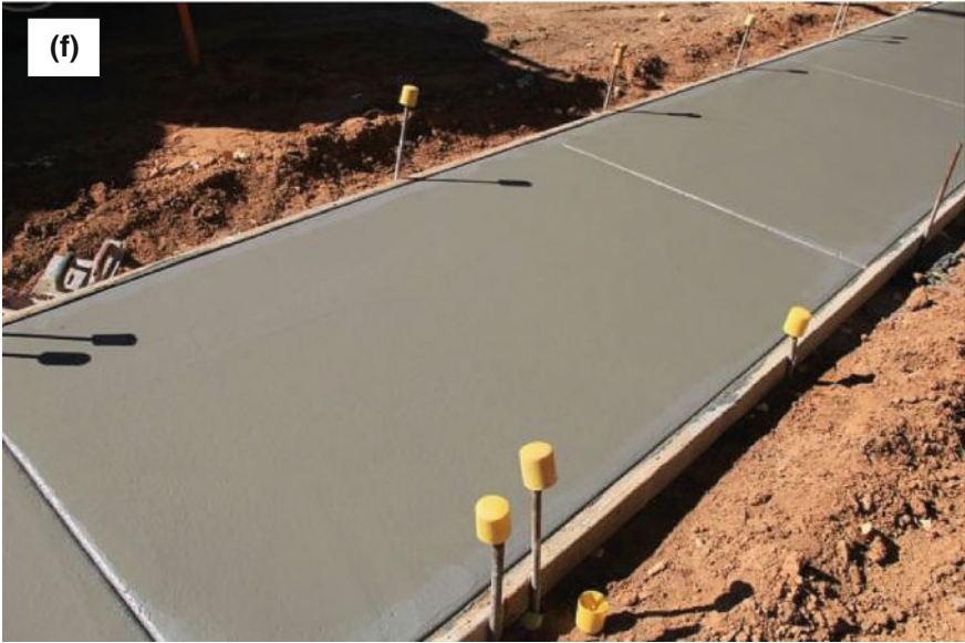
Finished footpath in the fresh stage
