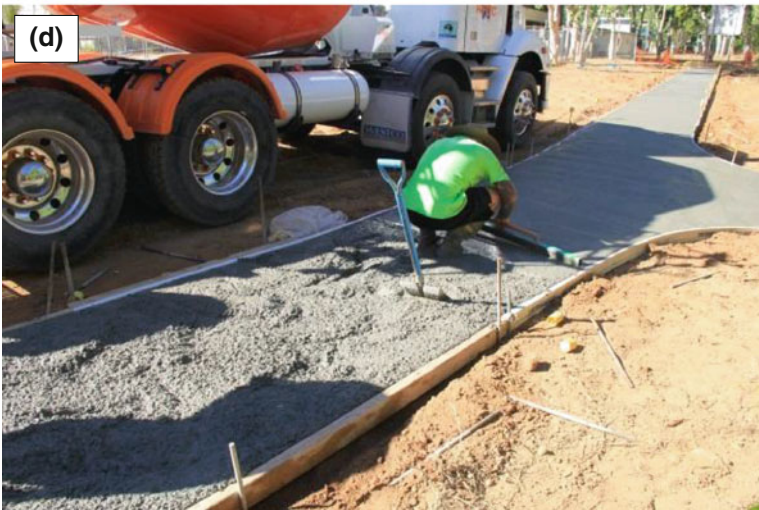
Smoothing the surface of footpath
