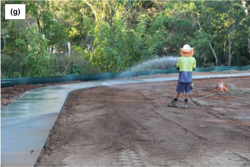
Water spraying for curing fresh concrete footpath
