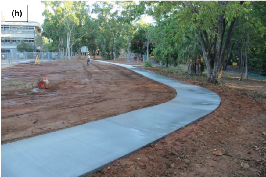
Footpath ready to use
