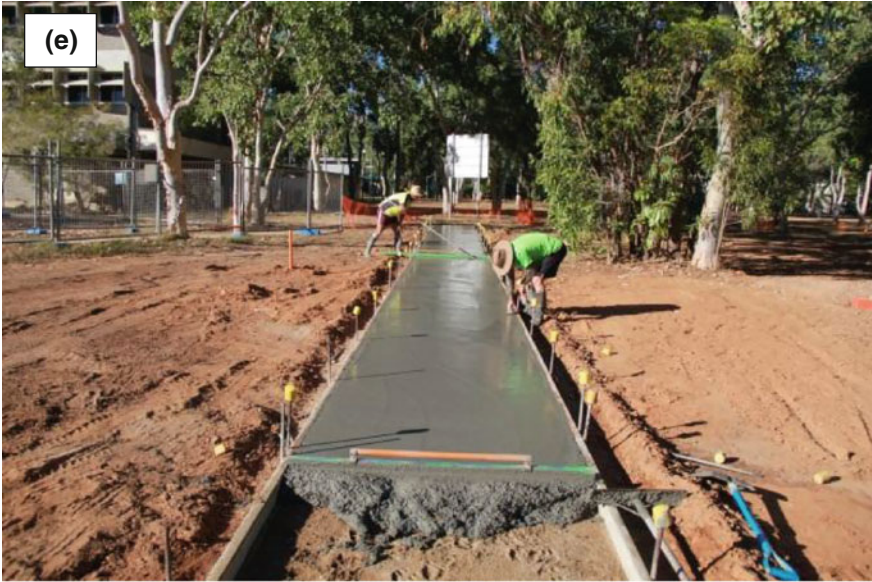
Edge smoothing and dummy joint
